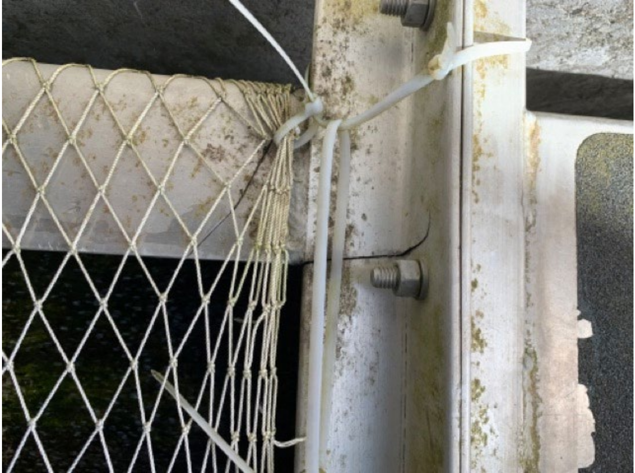
Crack on north ramp
